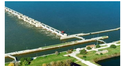
Mississippi River Lock & Dam
